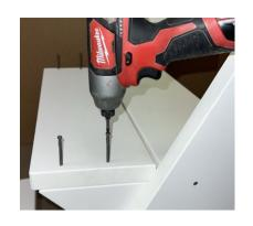
Screw down the front seat board second (the one with four holes), using four full length screws vertically.
