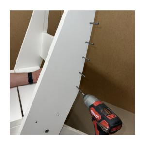
Screw down the back boards by attaching 3 on each side of each board through pre-drilled holes.
