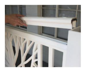
Secure top outer rail by applying adhesive along the length of the edges of the top support rail, OR by finish nailing through the side of the top outer rail into the top support rail.
